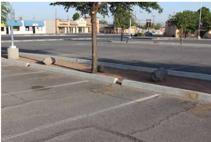
Figure 29: Curb cuts in a parking lot providing irrigation to median.
